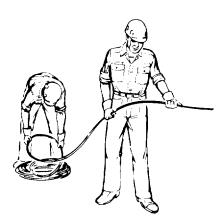
Figure 4-27. Incorrect Method of Unreeling Wire ROPe
